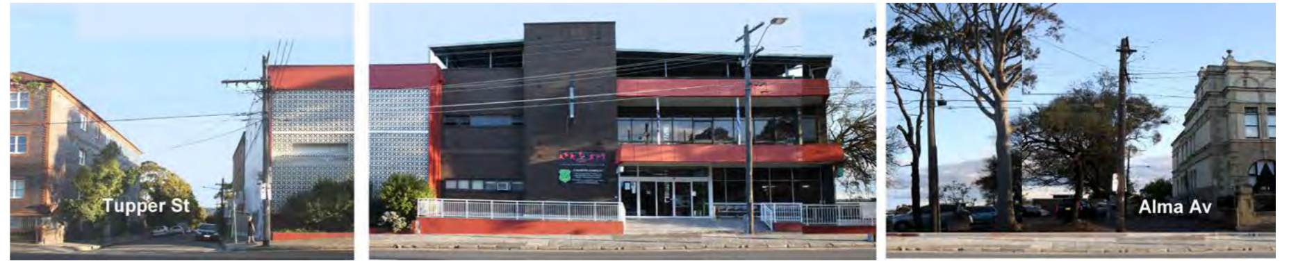
Existing Buildings Facing Stanmore Road
